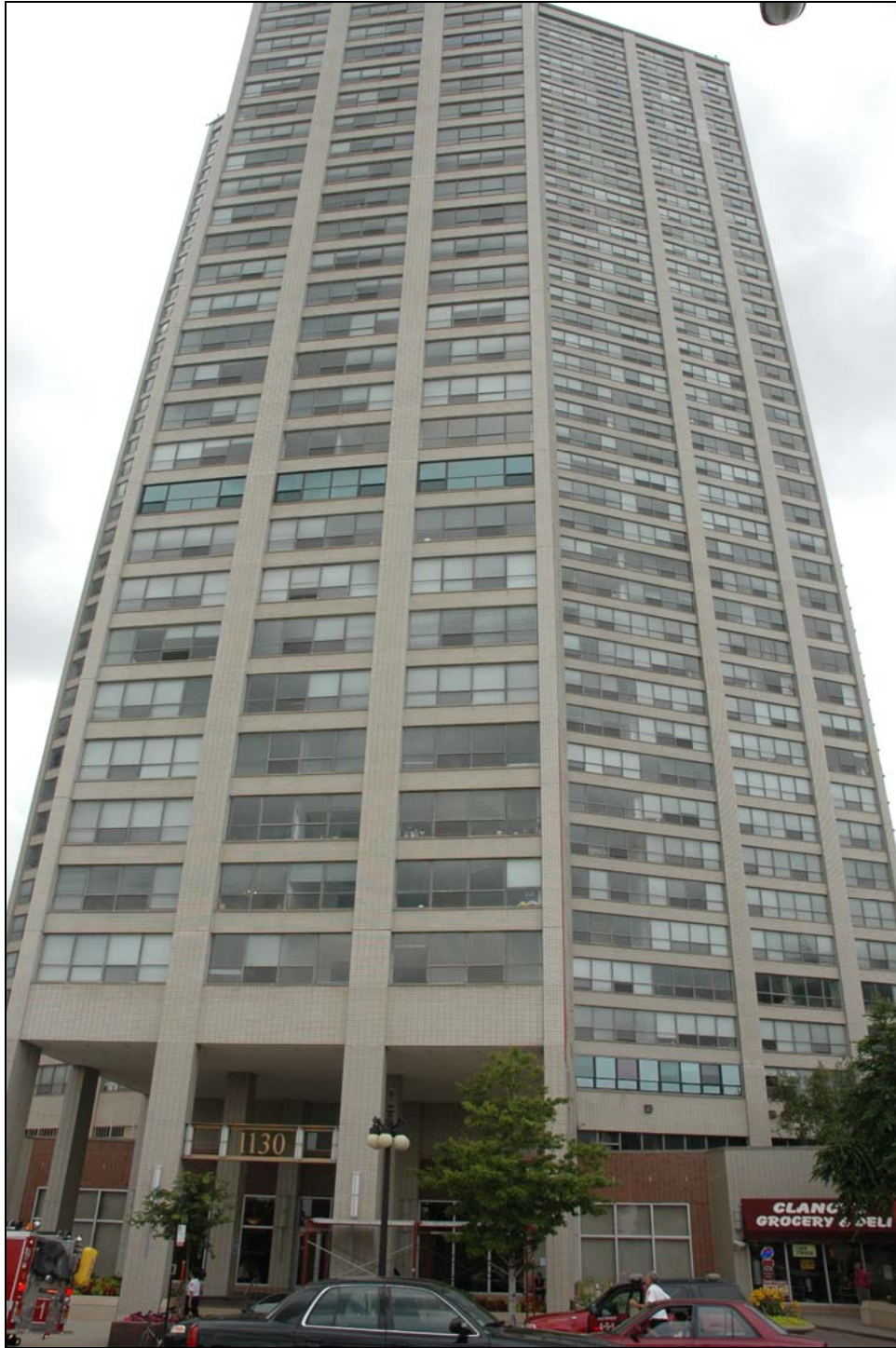
High-rise residential building at 1130 S. Michigan Ave.
