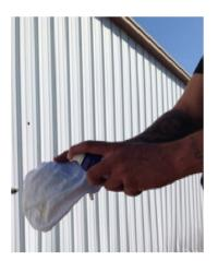
**Step Four:** Using a clean, dry cloth spray with Brake Parts Cleaner and wipe the entire exposed surface of the tube. **DO NOT** spray cleaner directly onto the tower itself or damage may occur. Depending on how dirty the section is, it may take several minutes to clean away the grime.
