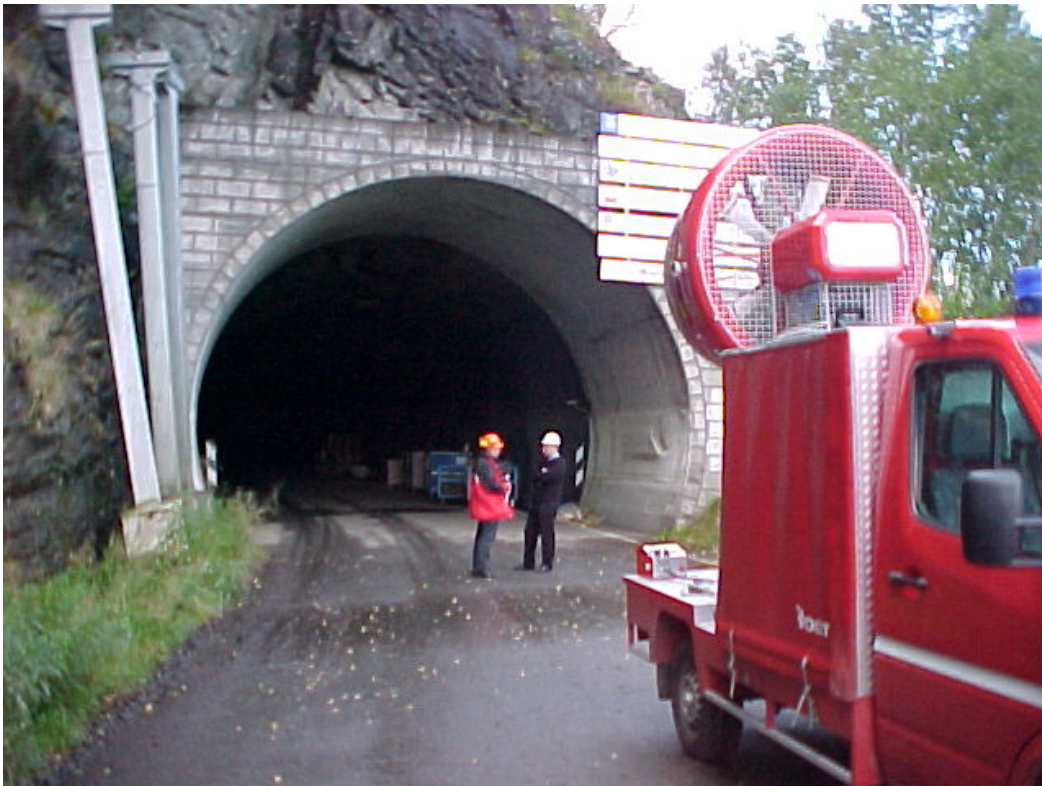
Truck mounted MVU positioned outside tunnel portal.
