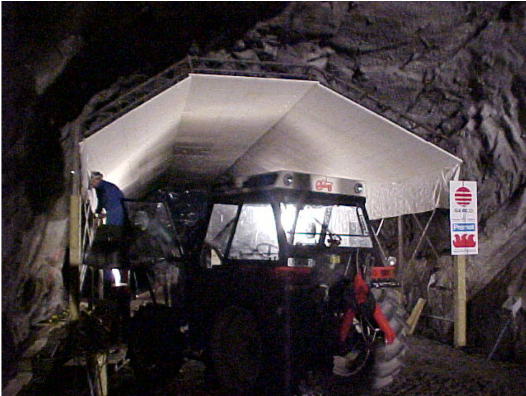
A heat-resistant shield was constructed inside the tunnel to protect the tunnel walls.
