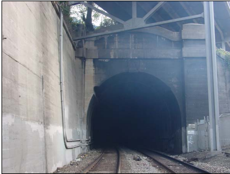
Figure 5: Smoke exiting the North Portal due to natural ventilation.
