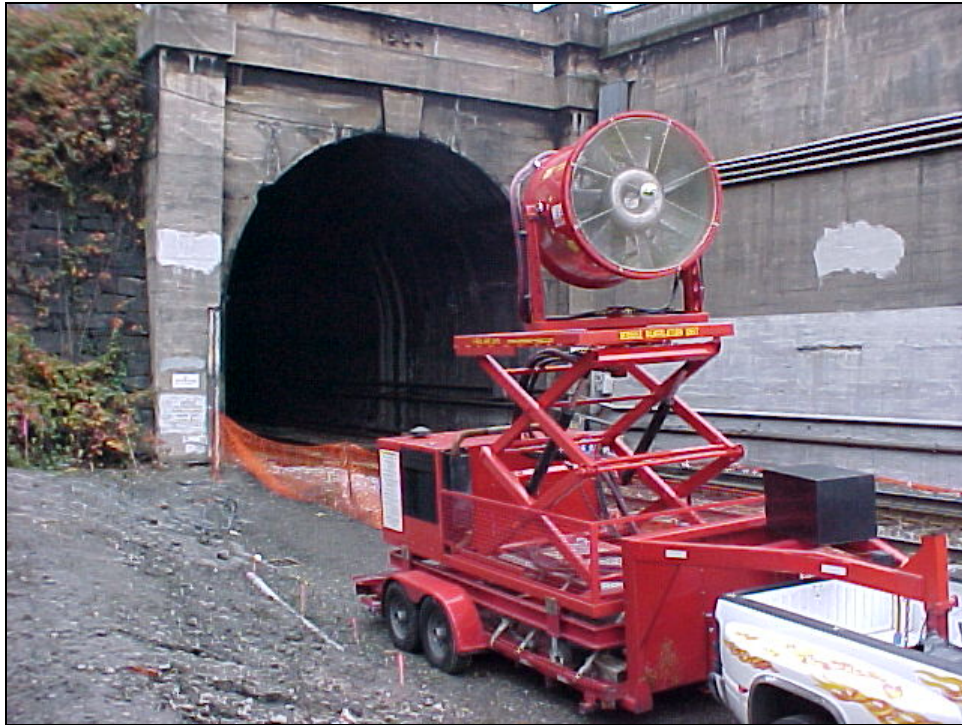
Figure 5: MVU elevated and aimed at center of tunnel bore
