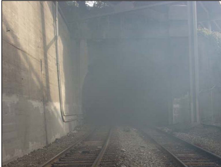
Figure 7: Smoke exiting the North Portal during PPV.
