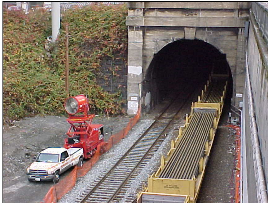
Figure 4: MVU Positioned at South Portal
