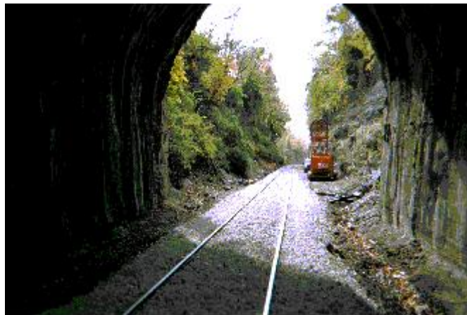
View From Inside Tunnel of MVU
