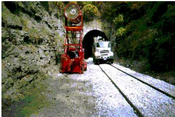
MVU Positioned in Front of Tunnel Portal
